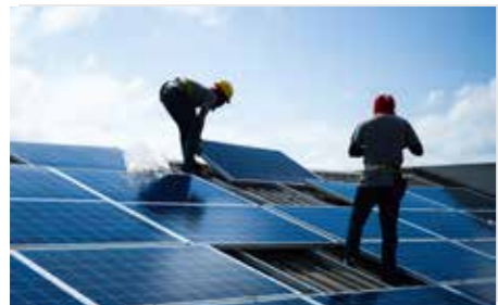
3. Safaga Port Project in Egypt, 1,000 kWp
