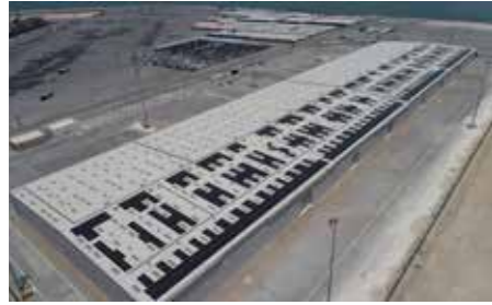
1. SouthQuay Warehouse 1 & 2 1,200 kWp
